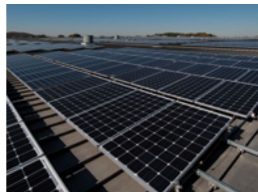
SOLAR ARRAY AT PLANT 15, CARTERSVILLE, GA
