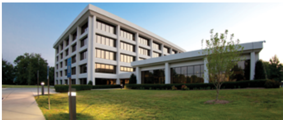
SHAW INDUSTRIES HEADQUARTERS IN DALTON, GEORGIA
